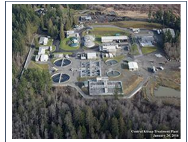
Central Kitsap Treatment Facility
