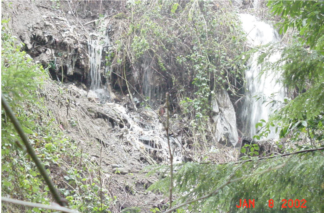
Photo No. 2 – Water and Waste Material Cascading Down the Exposed Face of Gorst Creek Landfill, 2002
