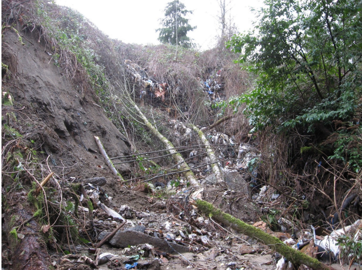
Photo No. 3 – Exposed Face of Gorst Creek Landfill after another Slide Event, 2007
